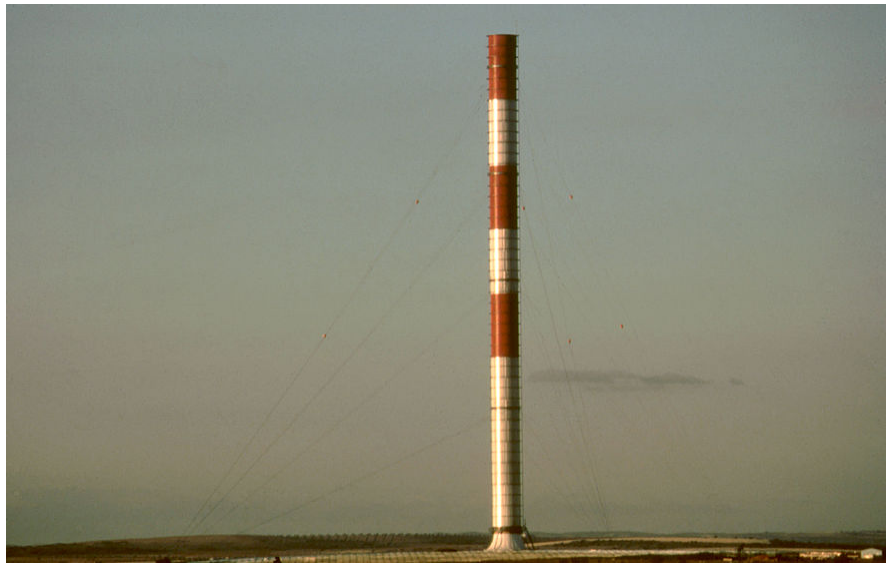
SUT powerplant prototype in Manzanares, Spain, seen from a point 8 km to the South
