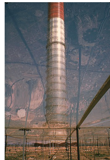
Manzanares Solar Chimney viewed through the polyester collector roof
