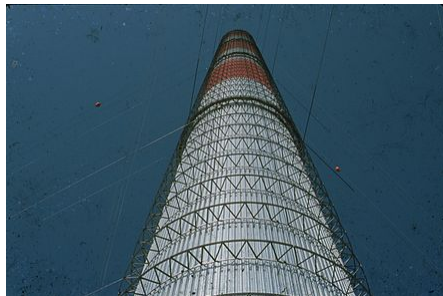
Manzanares Solar Chimney - view of the tower through the collector glass roof
