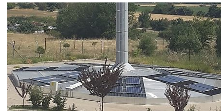
Solar towers can incorporate photovoltaic (PV) modules on transpired collectors for additional day time output and the heat from PV array is utilised by the solar tower
